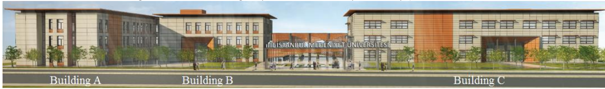
Figure 1. View of the building complex of Istanbul Medeniyet University. (Self-Elaboration).
