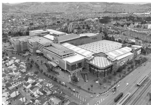
Centro Comercial Centro Mayor
