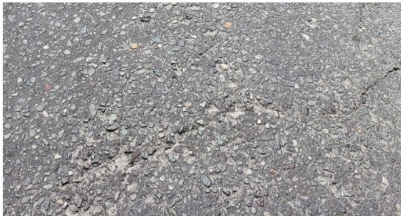
Figura 11. Surface damage for CDD=74.112 °C-days
